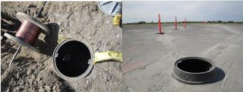
Above is a new “pull pit” and grounding wire as well as locations for the new runway end lights.
