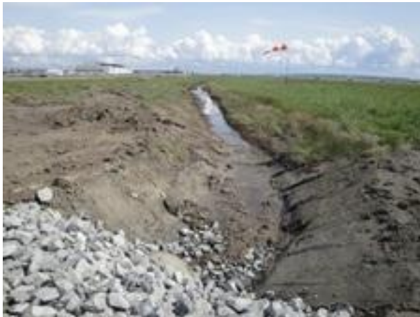
Drainage parallel to RW 07
